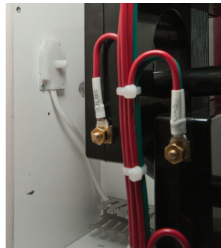
Examples of appropriate point sensor installation.
