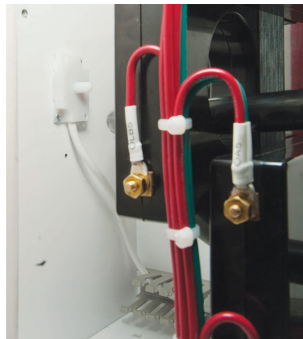
Examples of appropriate point sensor installation.
