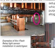
setup or configuration, which can defeat the purpose of the device altogether. A few Arc-Flash
